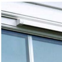
**Ventilation** - Vents can be fitted to the top rail of top sash. If fitted slide the cover sideways to open the vent to the desirable position. Care should be taken that the bottom sash does not contact the vent as this may cause damage to the internal vent cover.
