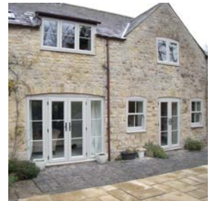
1990's timber framed double glazing replaced with PVC-U in a more appropriate design and traditional colour to enhance the property.
